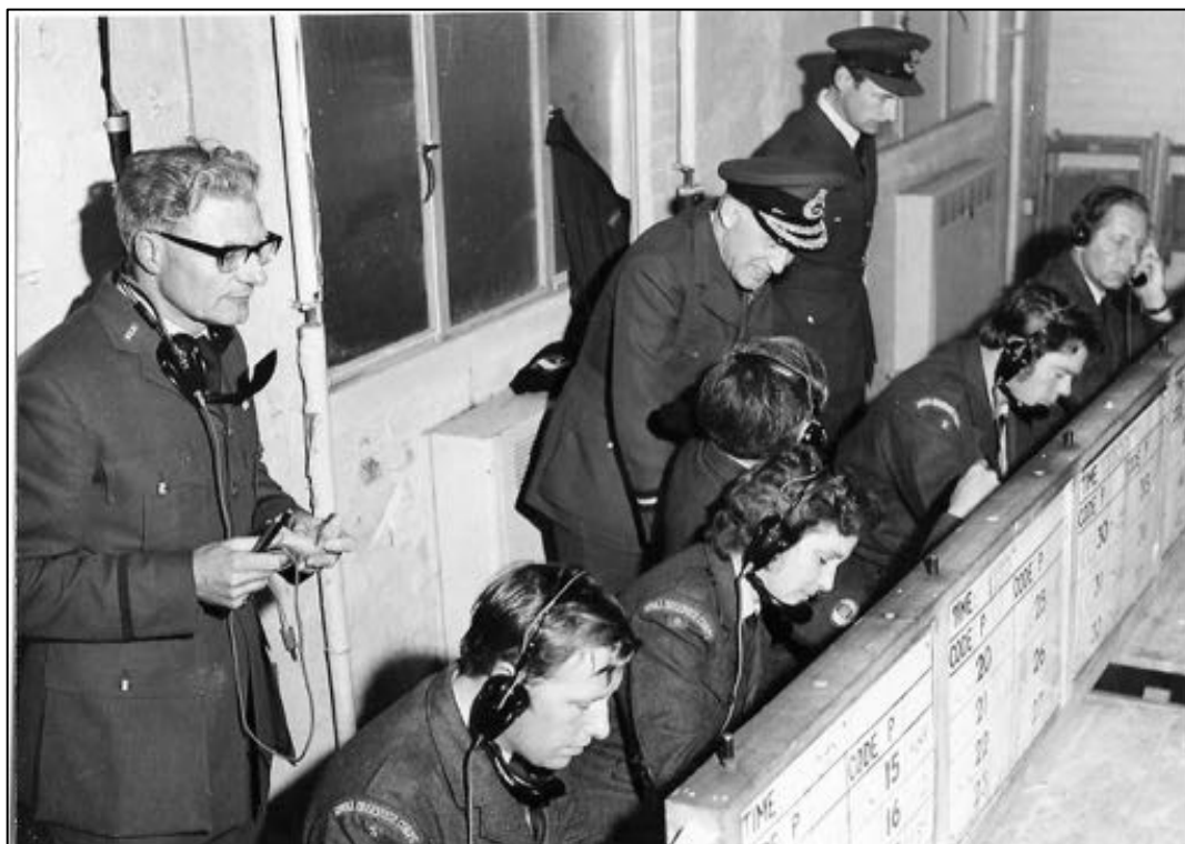
The above photo shows an ROC Ops Room
