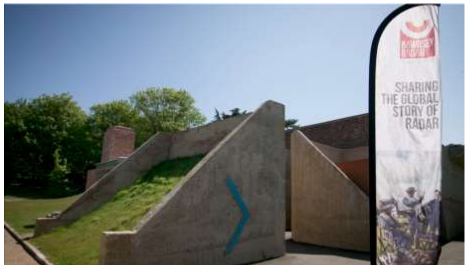
The Transmitter Block today
