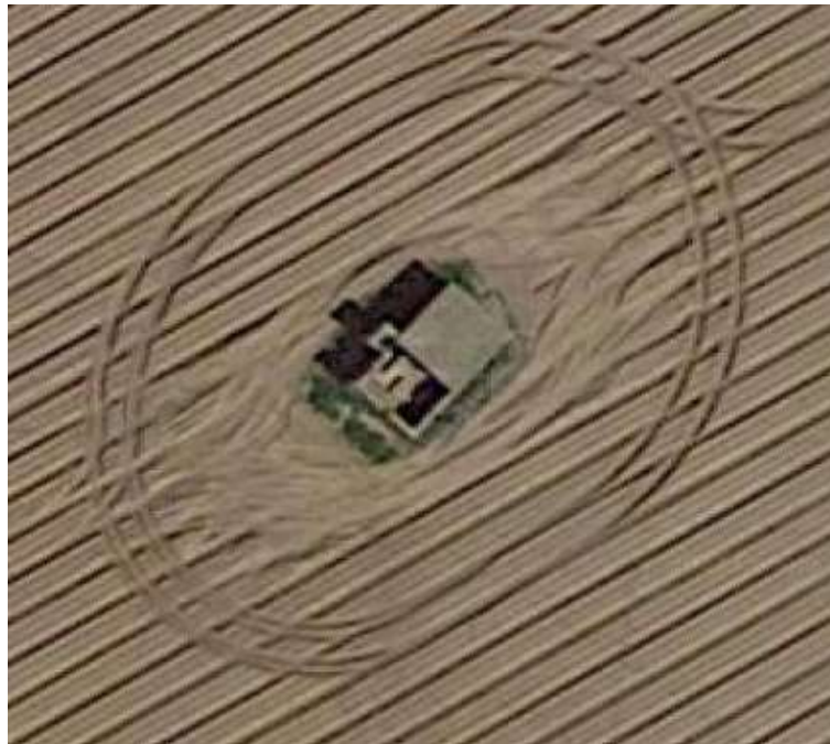
Figure 1; Aerial view of combined Anti-Aircraft gun site and pillbox south of Howlett Way, Trimley, part of the 1940 defences against invasion by airborne landings on the Deben levels. The landowner (Trimley Estates) reports that they will preserve the pillbox when the area is developed for housing.
