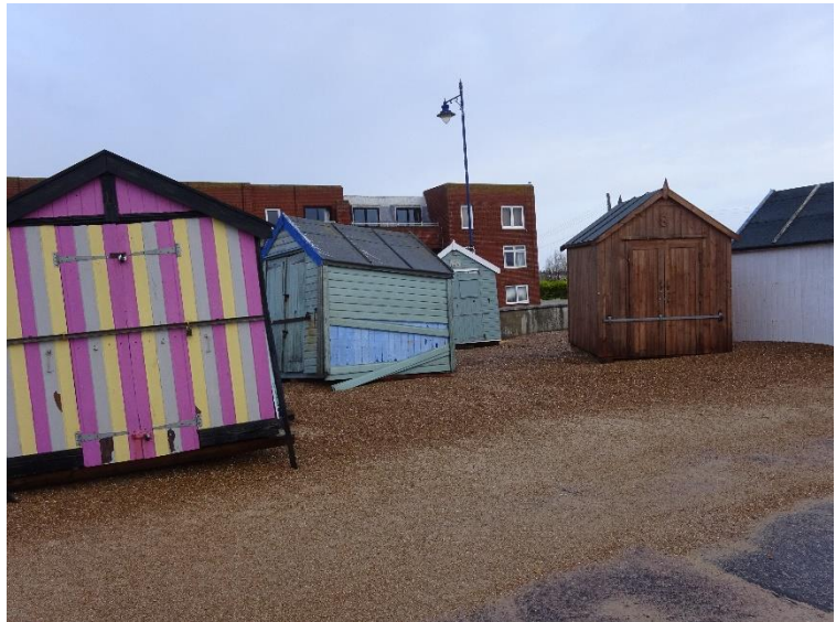
Some of the Damaged Beach Huts
