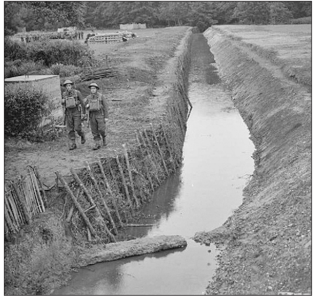
Figure 1 A typical Anti Tank Ditch
